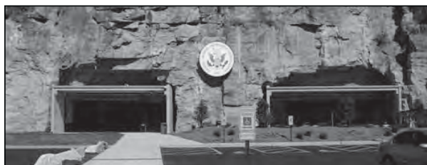
The development of Rock City in Valmeyer continues to attract prestigious records storage and warehousing clients, among them the National Archives and Records Administration. The agency employs some 150 people and stores more than 2.5 million cubic feet of records there.
