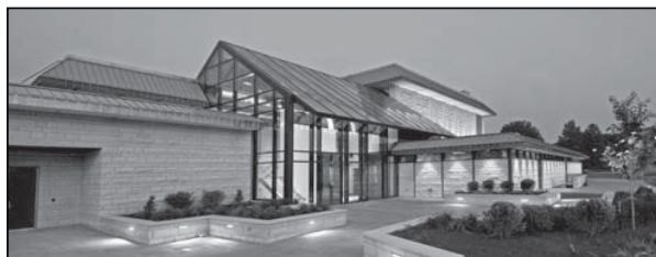
Contegra completed a $10.5 million renovation of Hatheway Hall at Lewis & Clark Community College in 2011.
