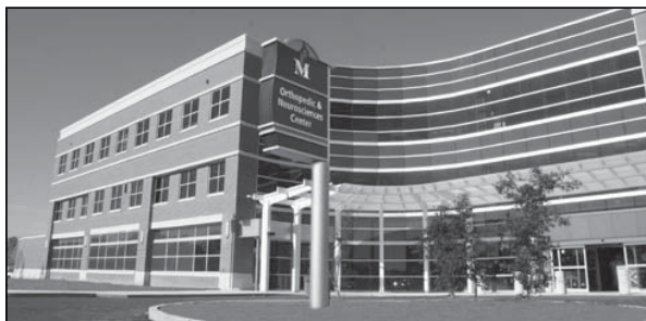
One of HCS' projects in the healthcare sector that reached completion in late 2011 was the Orthopedic and Neurosciences Center at Memorial Hospital in Belleville.
